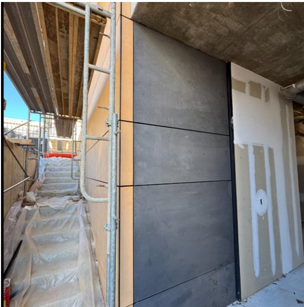
Installing exterior cladding.
