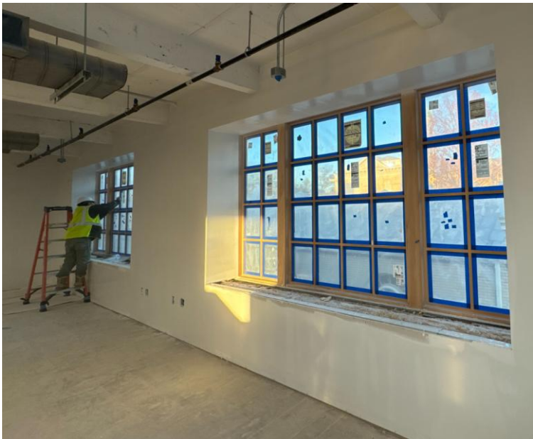
Finishing interior walls and prepping for paint.
