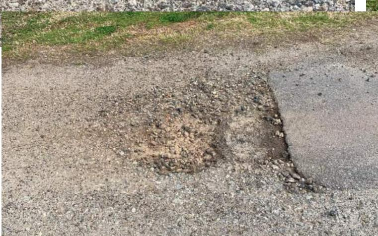
Failing subgrade and poor drainage are causing portions of the roadway to fail
