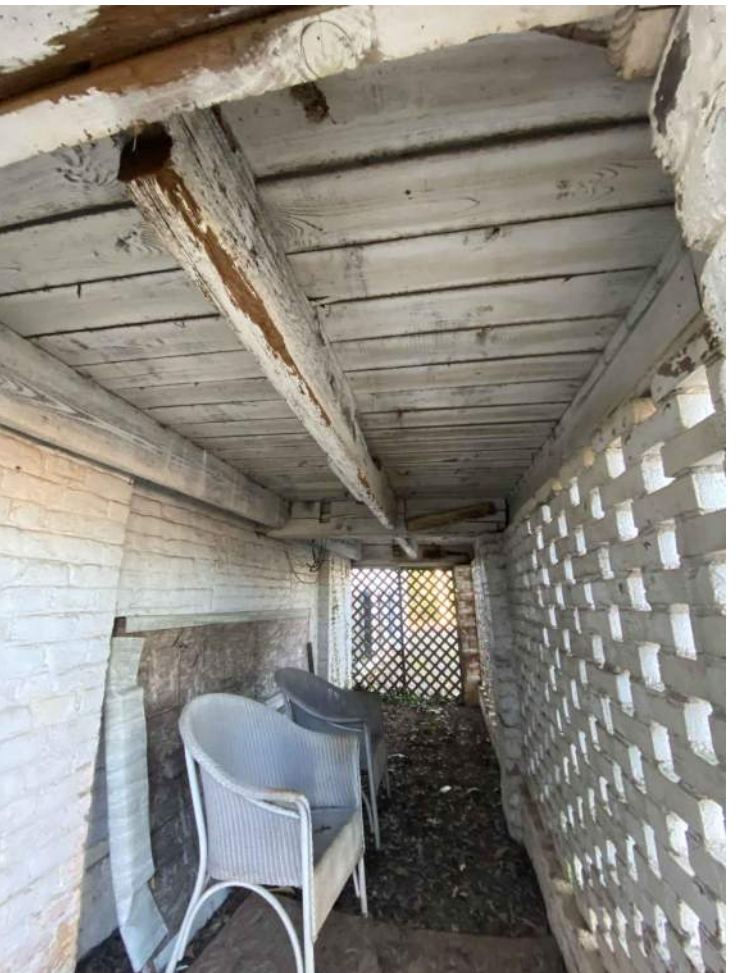
EXISTING FRAMING UNDER NORTH PORCH
