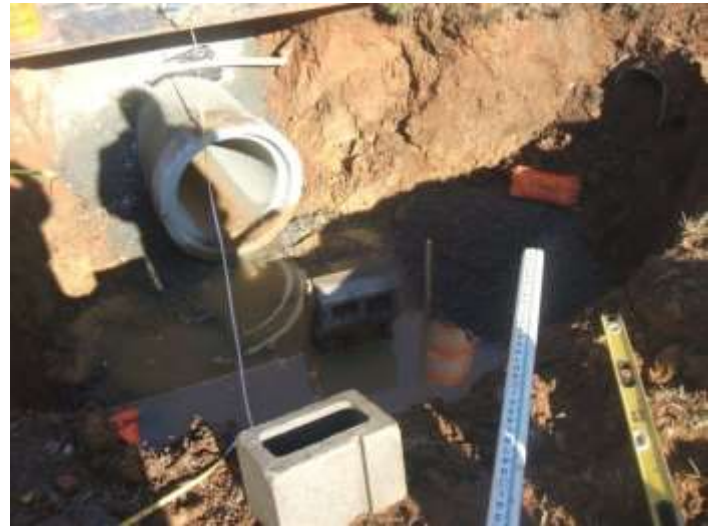
After – Stormwater Pipe
