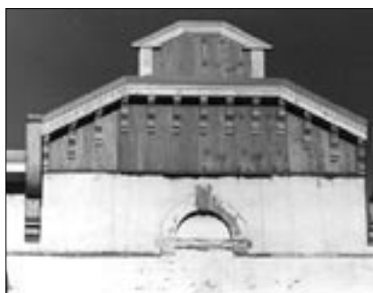
Reconstructing missing details using sufficient information is encouraged, this can be obtained from a historic photograph or investigation of physical evidence.
