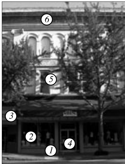
Typical storefront features include: 1) bulkhead, 2) display windows, 3) sign band, 4) recessed entry, 5) upper-story windows, and 6) cornice.
