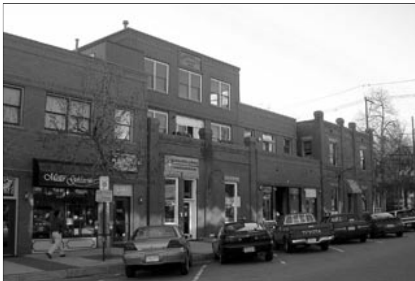
A roof addition should be set back from the primary, character-defining facade, to preserve the perception of the historic scale of the building. (Boulder, CO)
