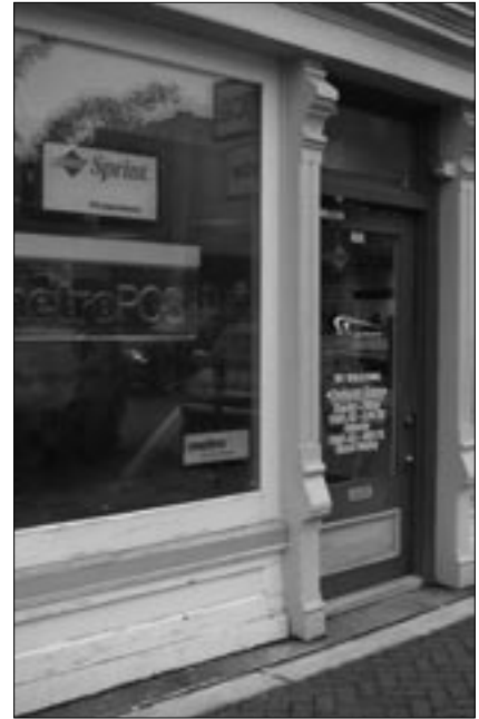
The bulkhead pictured beneath this display window includes appropriate historic details.
