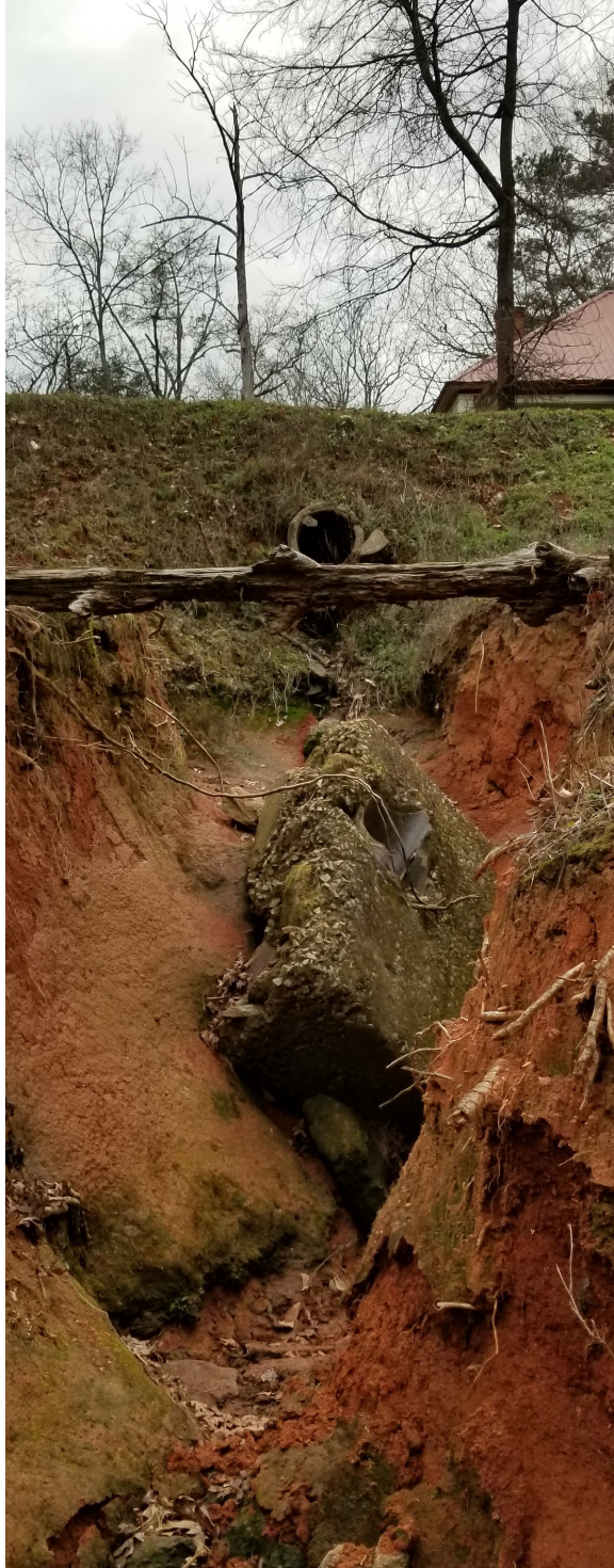
One of several stormwater infrastructure blow outs.
