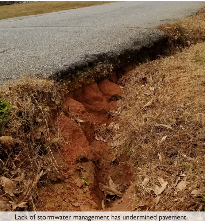
Lack of stormwater management has undermined pavement.
