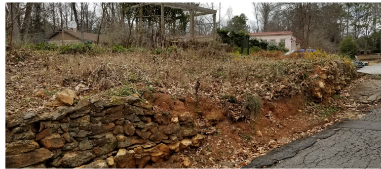
Improperly built stone retaining walls are crumbling throughout the park.
