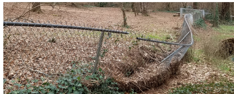
Heavy erosion in the dog park has created structural failures along the fenceline.
