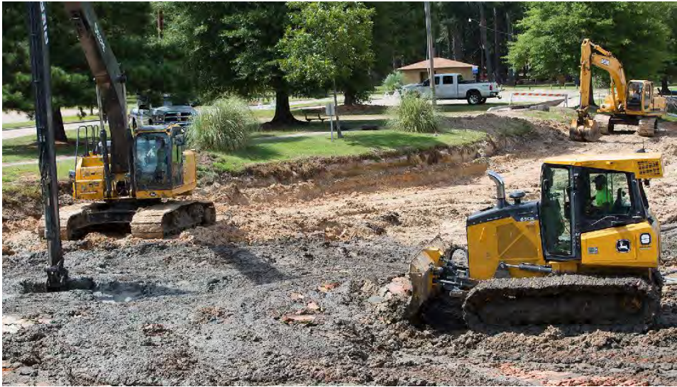
Typical mechanical pond dredging operations
