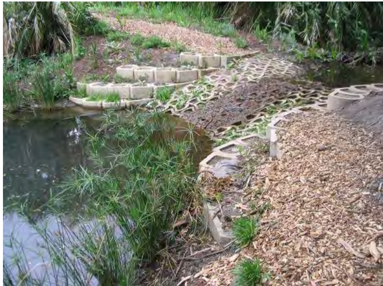
Concrete revetment at tributary entrance
