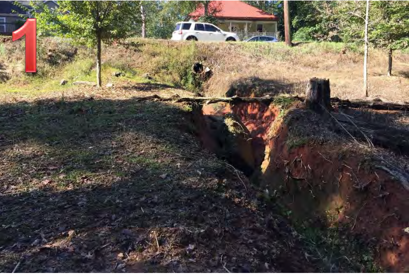
Mass wasting at outfall, facing West towards Lumpkin St.
