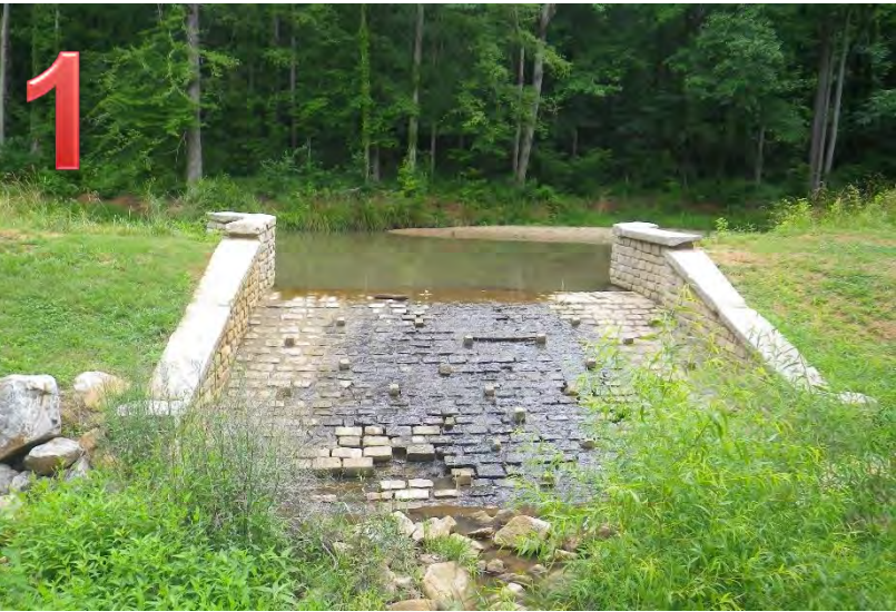
Existing deteriorating forebay outfall, facing NE
