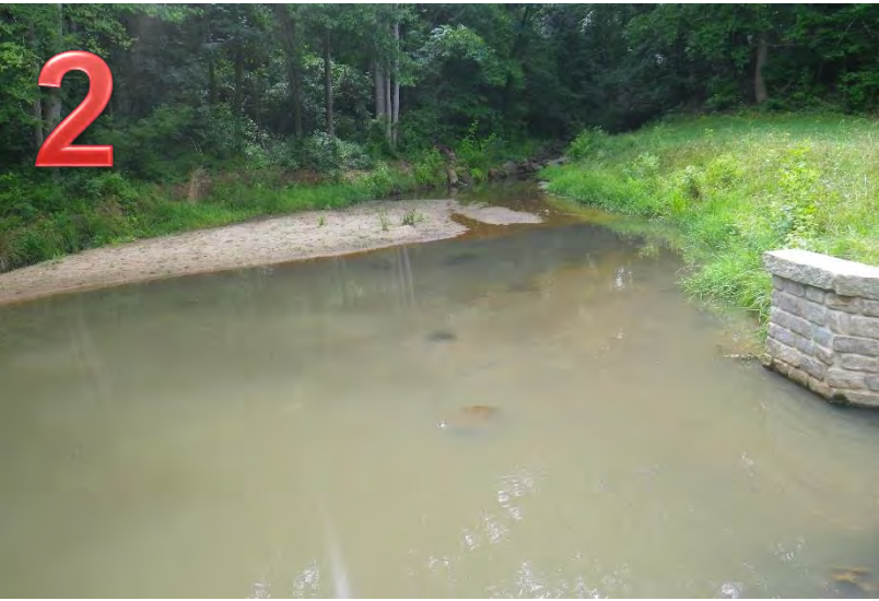
Forebay accumulating sediment, facing NE
