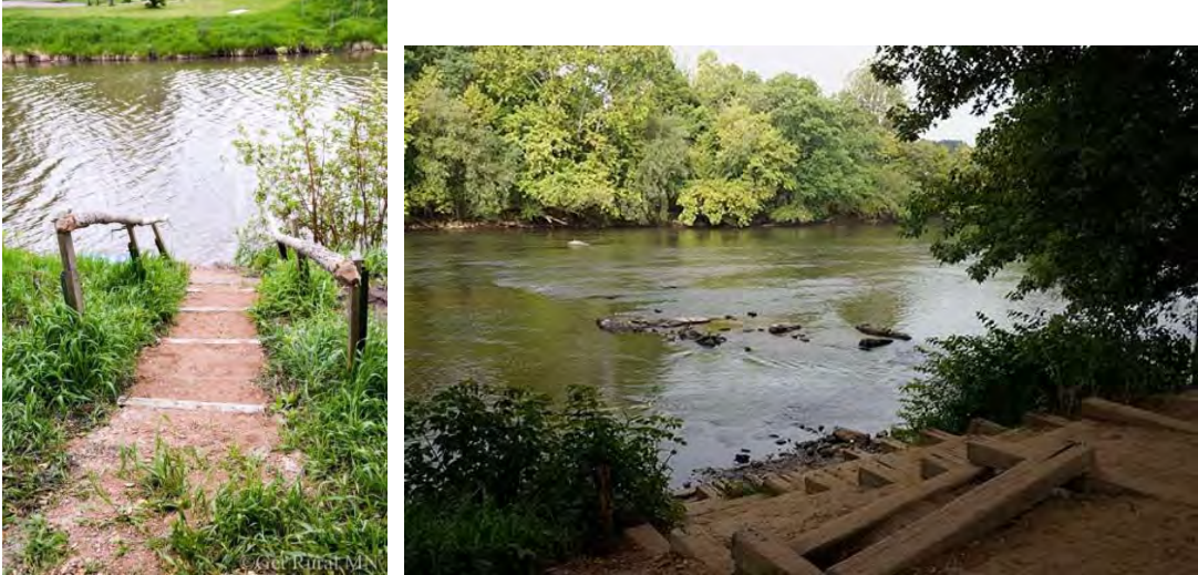
Example river access paths with stabilized banks
