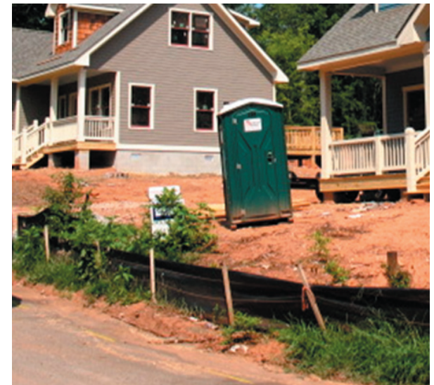
Figures 75 & 76 - Without regular maintenance and upkeep, graded sites associated with infill construction projects contribute to erosion sediment in stormwater flows. The trail of red clay along the street surface above demonstrates how, even with silt fencing in place, some degree of erosion on graded sites is inevitable.
