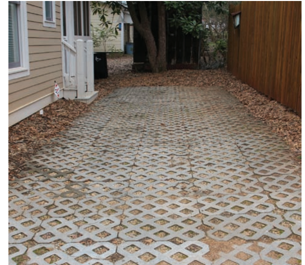
Figure 74 - Pavers designed to allow water filtration provide an attractive and beneficial surface for residential parking, but they are included in the lot coverage area.
