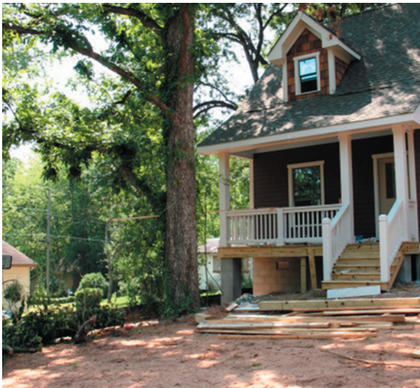
Figure 79 & 80 - Grading, structure placement and a general lack of protective measures within the drip line of this mature hardwood (left) do not bode well for the tree's survival. On a previously undeveloped lot, the mature pecan (right) is left with a fraction of its root surface area after recently completed construction.
