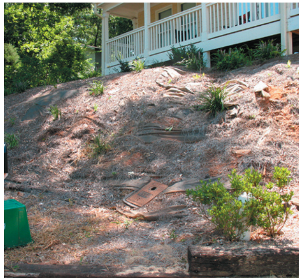
Figures 75 & 76 - Without regular maintenance and upkeep, graded sites associated with infill construction projects contribute to erosion sediment in stormwater flows. The trail of red clay along the street surface above demonstrates how, even with silt fencing in place, some degree of erosion on graded sites is inevitable.
