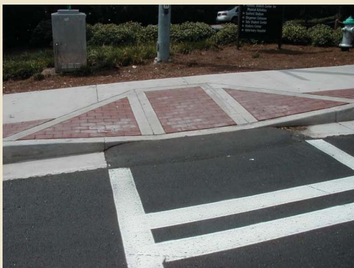
Pedestrian ramp with brick pavers and standard striped crosswalks
